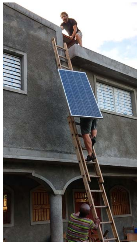
Installing solar panels on a school in Duchity, Haiti
